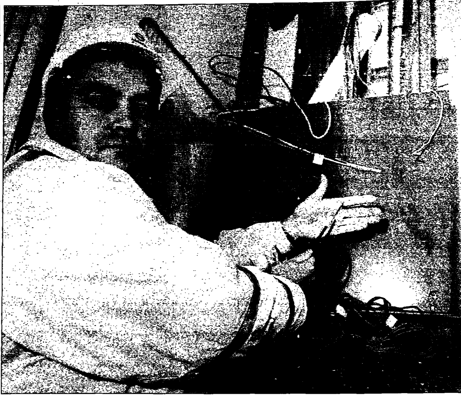
Paul Gover, station delivery manager for the Jubilee Line, with some of the vandalised cables at the London Bridge station on the Jubilee Line
